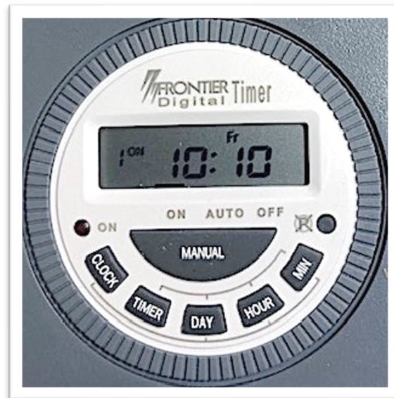
Time clock front panel. Note the "Manual ON-AUTO-OFF" button and cursor.
